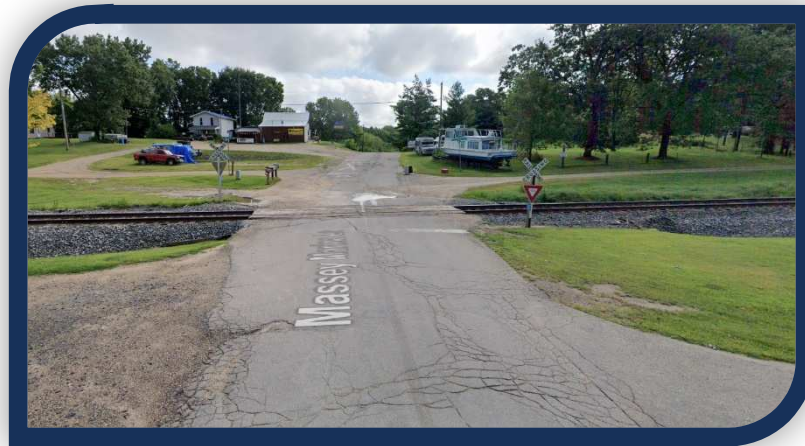
Figure 18 – Massey Marina Lane Crossing
